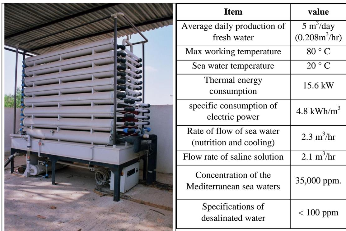
**Figure 15: A view of the MSF Desalination unit and its technical specification.**
